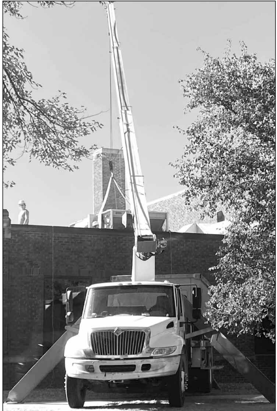
A large crane delivers a new HVAC unit to the South Barber Elementary School. The cost of this project is about $400,000.
